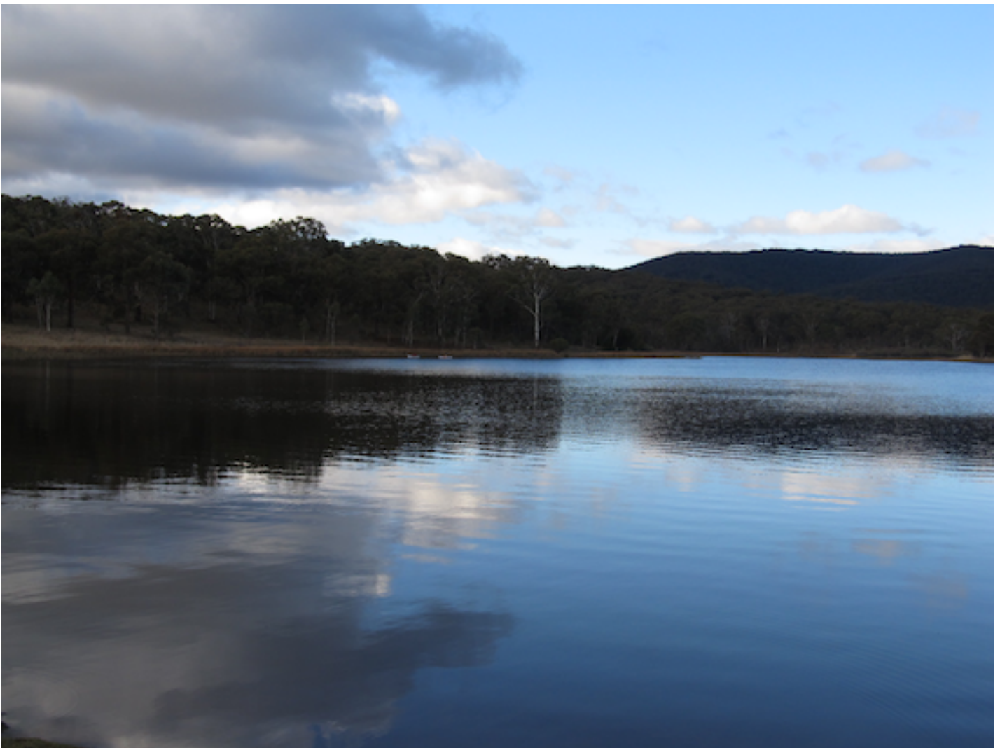
Dumaresq Dam near Armidale NSW Image: M. Hitchcock
